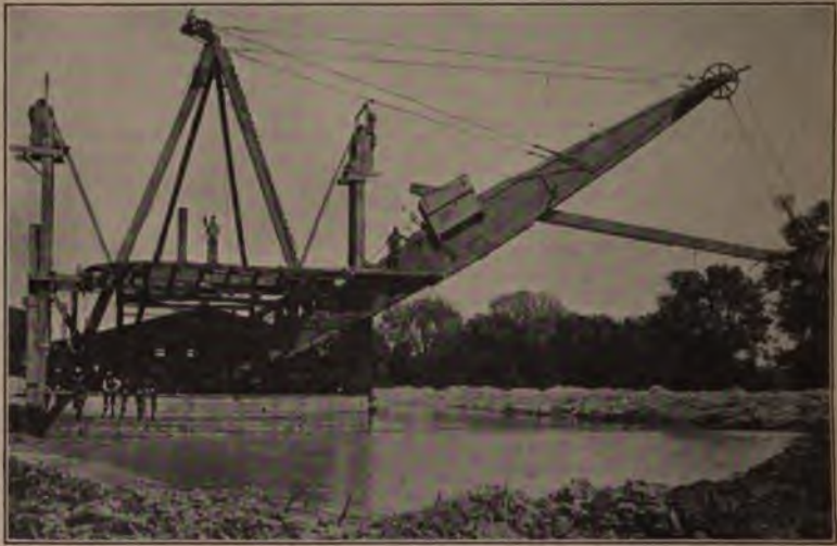
Floating Dipper Dredge Excavating Drainage Ditch.
